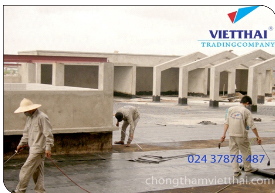
Construction of torched on membrane
