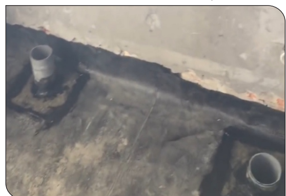
Finish the neck of the pipe and the Baseline corner
